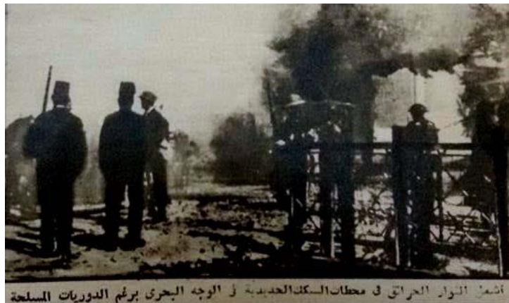
Figure (1) Encroachments on the rails, and locomotives of the railway between Tala and Tanta, (Courtesy of Samir el Ghazuli).
