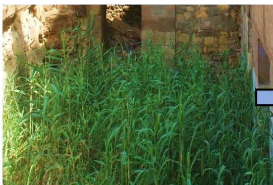
(a) Current status of entrance.
